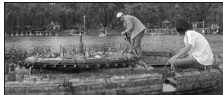
Taking measurements of the existing fountain facilities in the middle of Burnham Lake.
